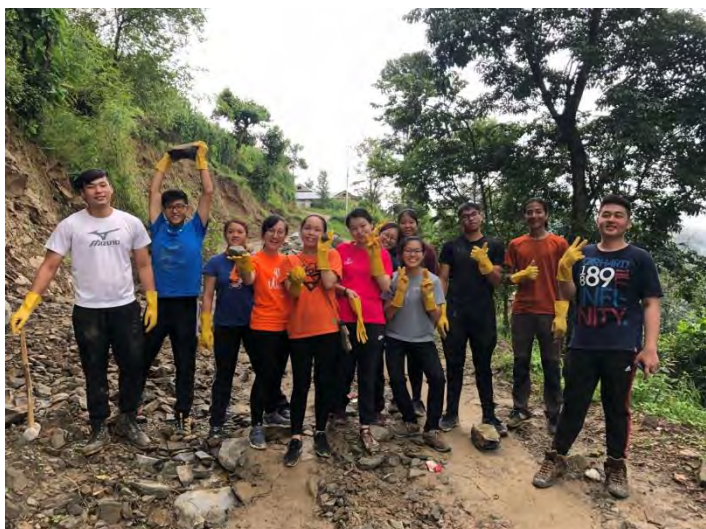
Roads were destroyed during earthquake. This made villagers difficult to go in and out of the village and might even get hurt. Participants helped reconstruct a new staircase.
